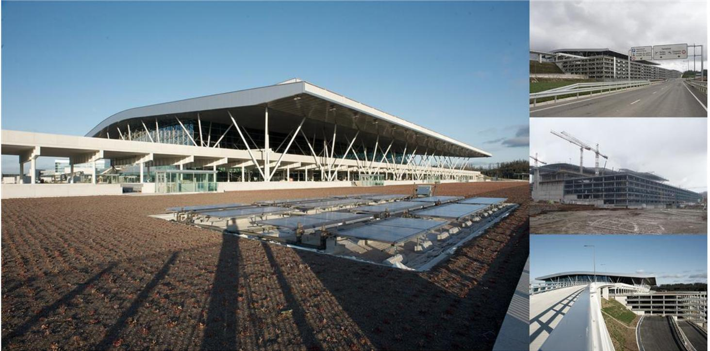
The car park building at Santiago Airport Terminal has surface area dimensions of 325.50m x 92.10m. It is a semi-below grade structure for vehicles, which has 5 basements plus a lower level dedicated to the installations. The spans between columns vary between one direction and another. On axis Y the span is 8.0m or 8.33m and on axis X the span is 8.33m.
